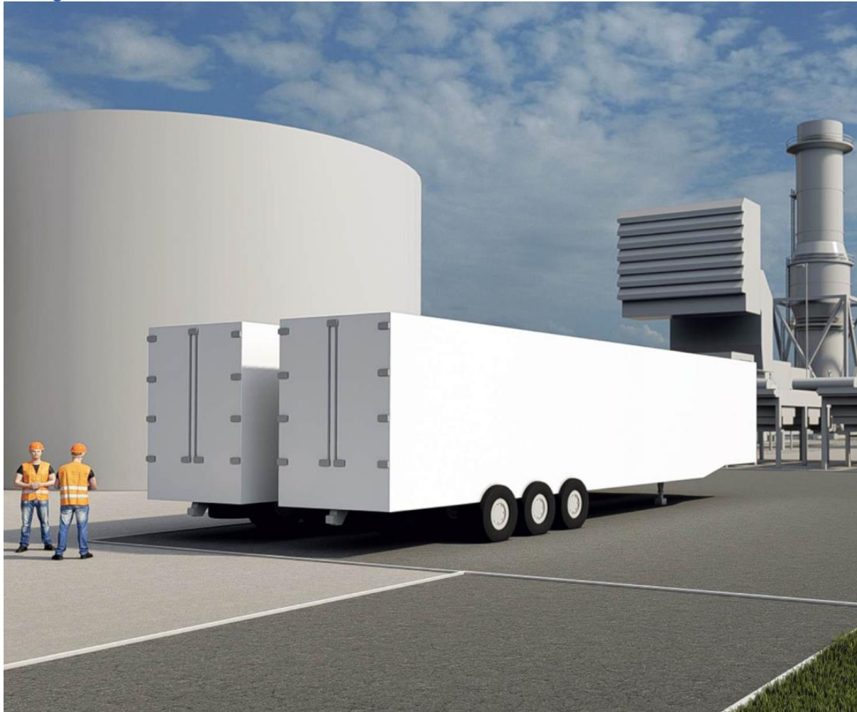
Figure 5.6: View of water treatment trailers, with storage tank within the ancillary compound in the left background, and the proposed gas turbines in the right background
